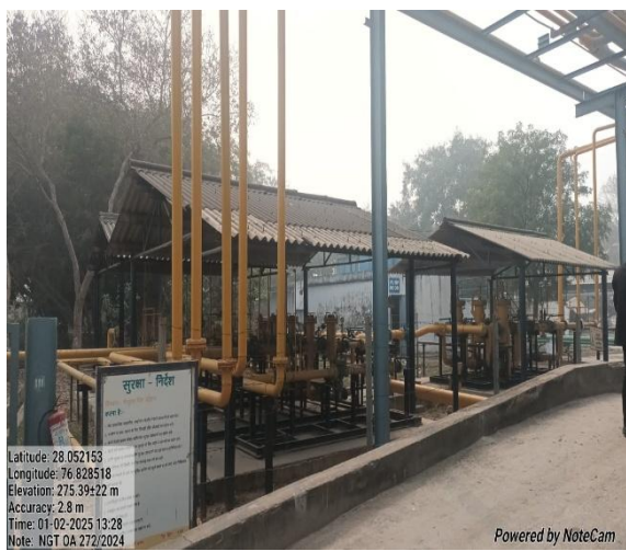
PNG station installed by GAIL in the premises
